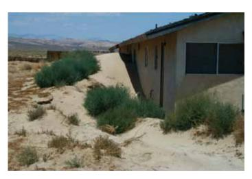
Figure 13: Rancho Seco residence has sand accumulation on the upwind side of the house.
