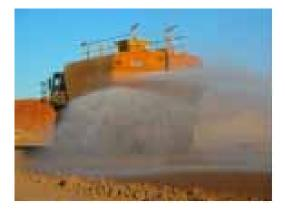
Figure 11: A water truck applies a chemical binder to the road.
