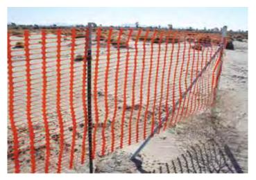
Figure 7: This 50% wind porosity fencing causes dust to deposit more on the downwind side of the fence.
